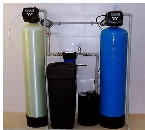
Fig. 2. Column granular filters to brighten the water and an activated carbon sorption filter
