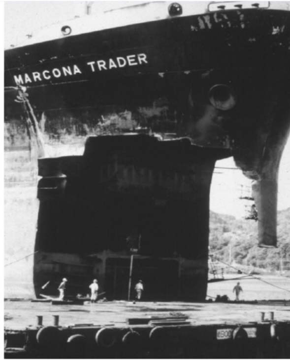
Fig. 3. Repair of damage to the fore end of the hull of the bulk carrier Marcona Trader [7]
