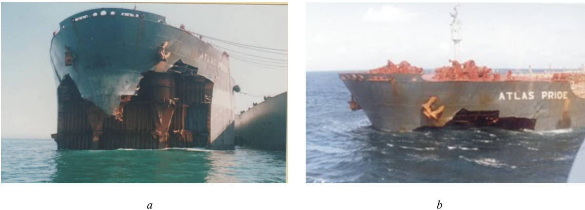
Fig. 1. Damaged bow end of the oil ore carrier Atlas Pride [5]: a – front view; b – side view
